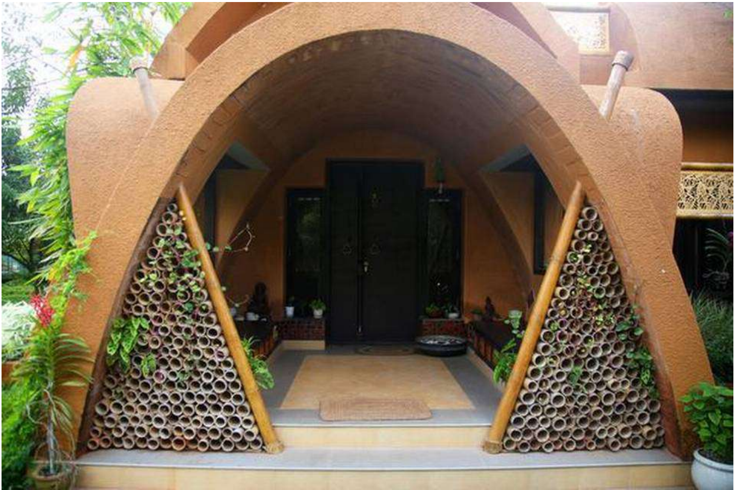
Porch with bamboo grills and the front door | Photo Credit: Aswin V.N.
